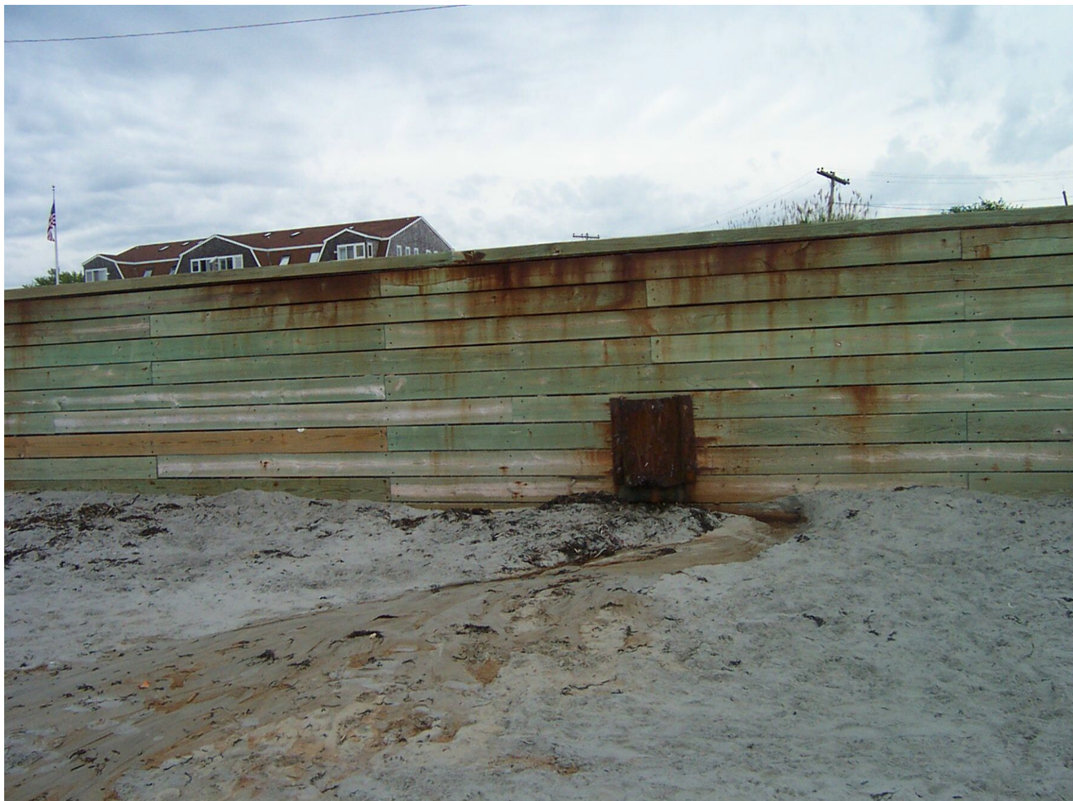
Figure 10. Photograph of outfall at base of the seawall along Goochs Beach showing liquid discharge. No rain events had occurred in the several days preceding this site visit. Image taken by P.A. Slovinsky, MGS, July 6, 2006.
